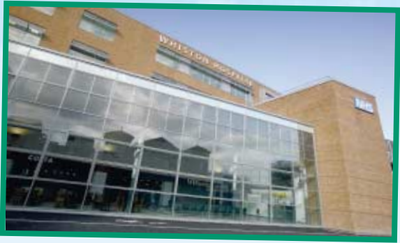
The old hospital reflected in the glass of the main atrium in the new Whiston Hospital
