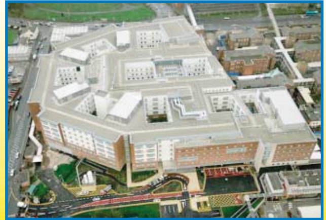
An aerial photograph of the new Whiston Hospital
