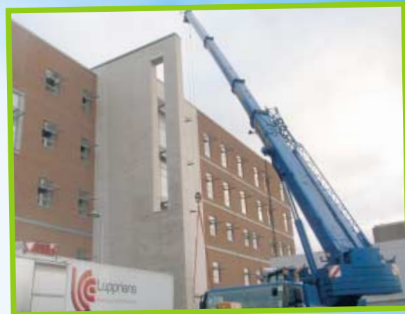
The big crane that lifted the magnet
