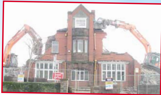
Demolition started on the old St Helens Hospital
