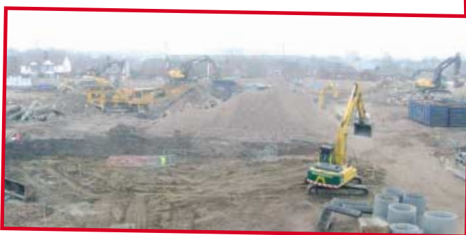
Demolition work in December 2008
