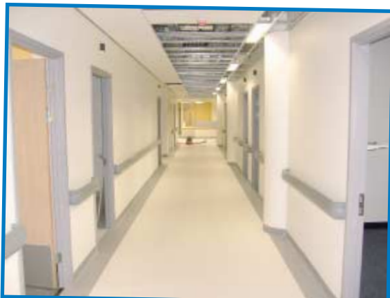
A new corridor at St Helens Hospital
