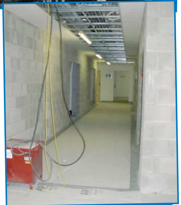
The flooring is down in the kitchens
