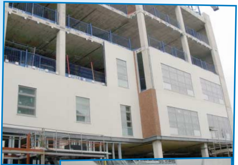
The new windows are installed at Whiston
